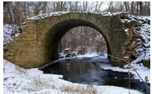
Old Stone Arch Bridge across Brown's Creek in Stillwater, MN
