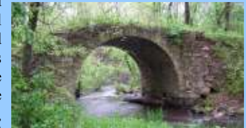
Historic Stone Arch Bridge over Brown's Creek – 2011 Stabilization Project Permitted through BCWD partnership
