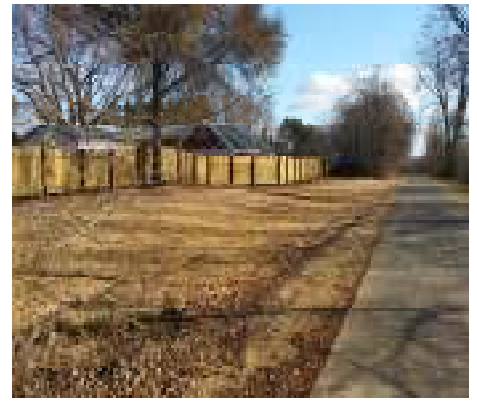
Just after construction (Oct 2014)
