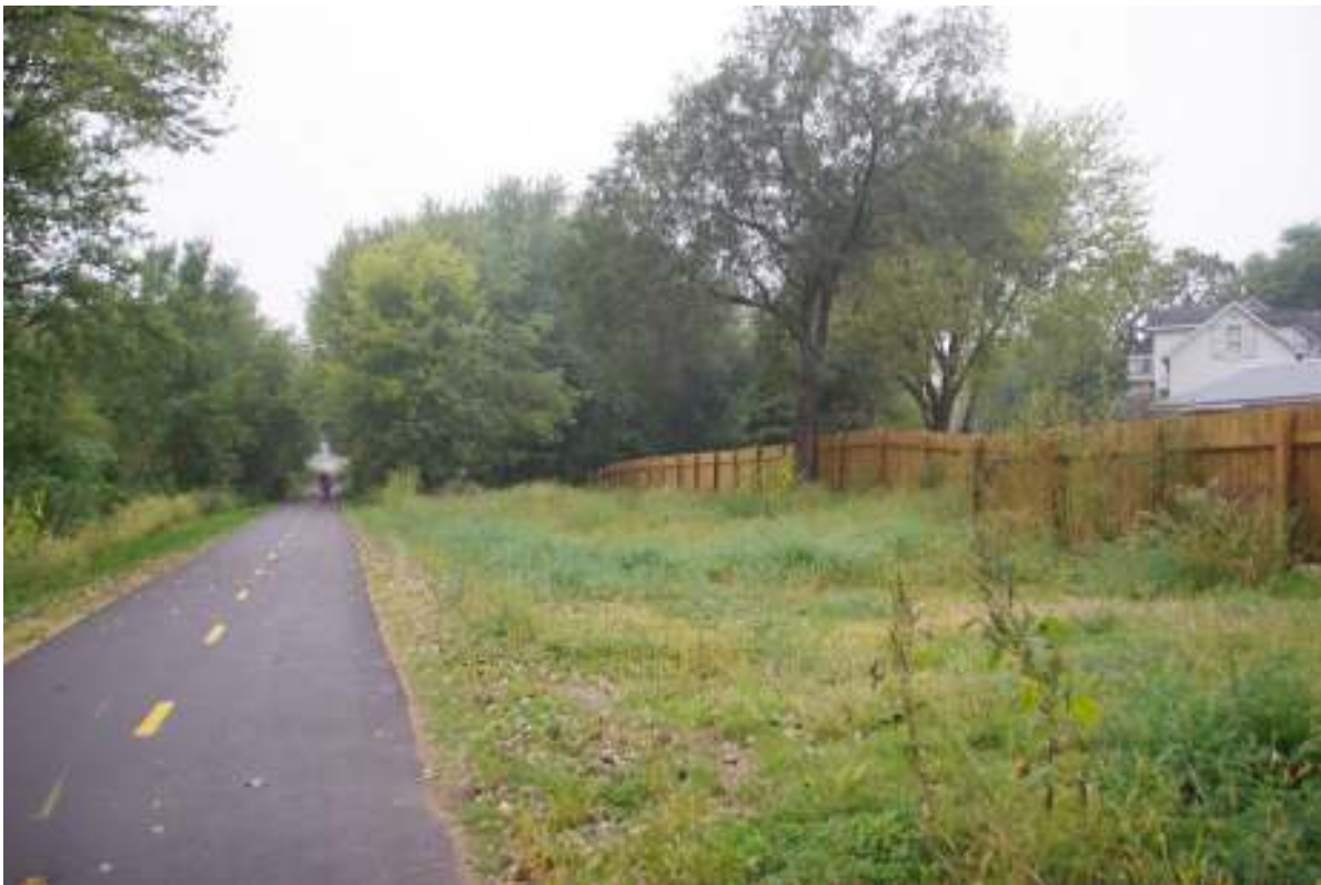
September 2015 - Brown's Creek water quality improvement project: site of an underground HDPE Water Quality Unit with associated inlet and outlet pipes and manhole structures within the DNR Trails Right-of-Way for sediment capture off of parking and drive lanes from Countryside Auto before entering an impaired trout stream.
