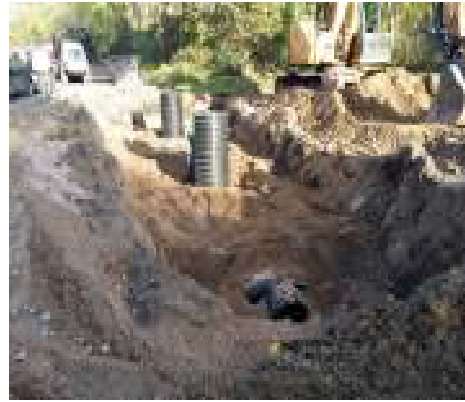
During Construction (Sept 2014)
