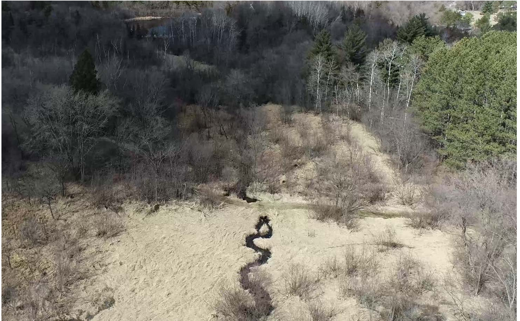
Twin culverts under a trail crossing downstream of 110 th St
