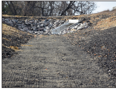
Side-water inlets, left and right , are part of the BDSWD's multipurpose drainage management work on Traverse County Ditch 35 supported by a Clean Water Fund grant from BWSR. The project has water storage, water quantity and water quality benefits. Work finished in fall 2022. Middle: In Redpath Township, Traverse County Ditch 35 outlets into Twelvemile Creek through a culvert. The ditch, seen here in October 2022, would usually contain water that time of year.
