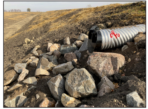
Side-water inlets, left and right , are part of the BDSWD's multipurpose drainage management work on Traverse County Ditch 35 supported by a Clean Water Fund grant from BWSR. The project has water storage, water quantity and water quality benefits. Work finished in fall 2022. Middle: In Redpath Township, Traverse County Ditch 35 outlets into Twelvemile Creek through a culvert. The ditch, seen here in October 2022, would usually contain water that time of year.
