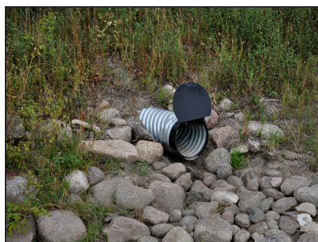
Left: Gently sloped sides are one element of a Traverse County Ditch 37 retrofit. The retrofit will help alleviate flooding in farm fields and improve water quality within the Bois de Sioux Watershed by allowing nutrient-carrying sediment to settle. Middle: Side-inlet culverts in the berm connect the ditch to the field. When the water level in the ditch is high, the pressure pushes a flap-gate shut. Water then remains on the field until the level in the ditch drops. Right: Check dams help to reduce the velocity within the ditch.
