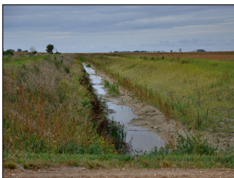
Left: Gently sloped sides are one element of a Traverse County Ditch 37 retrofit. The retrofit will help alleviate flooding in farm fields and improve water quality within the Bois de Sioux Watershed by allowing nutrient-carrying sediment to settle. Middle: Side-inlet culverts in the berm connect the ditch to the field. When the water level in the ditch is high, the pressure pushes a flap-gate shut. Water then remains on the field until the level in the ditch drops. Right: Check dams help to reduce the velocity within the ditch.
