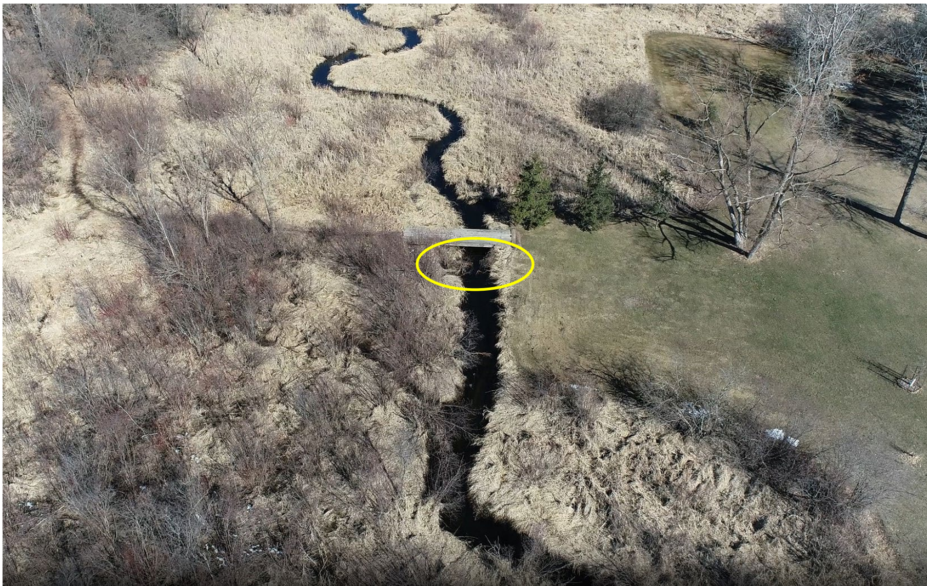
Wood bridge and location of old beaver dam (yellow oval) near private parcel west of 97 th St. N / downstream of the Gateway Trail
