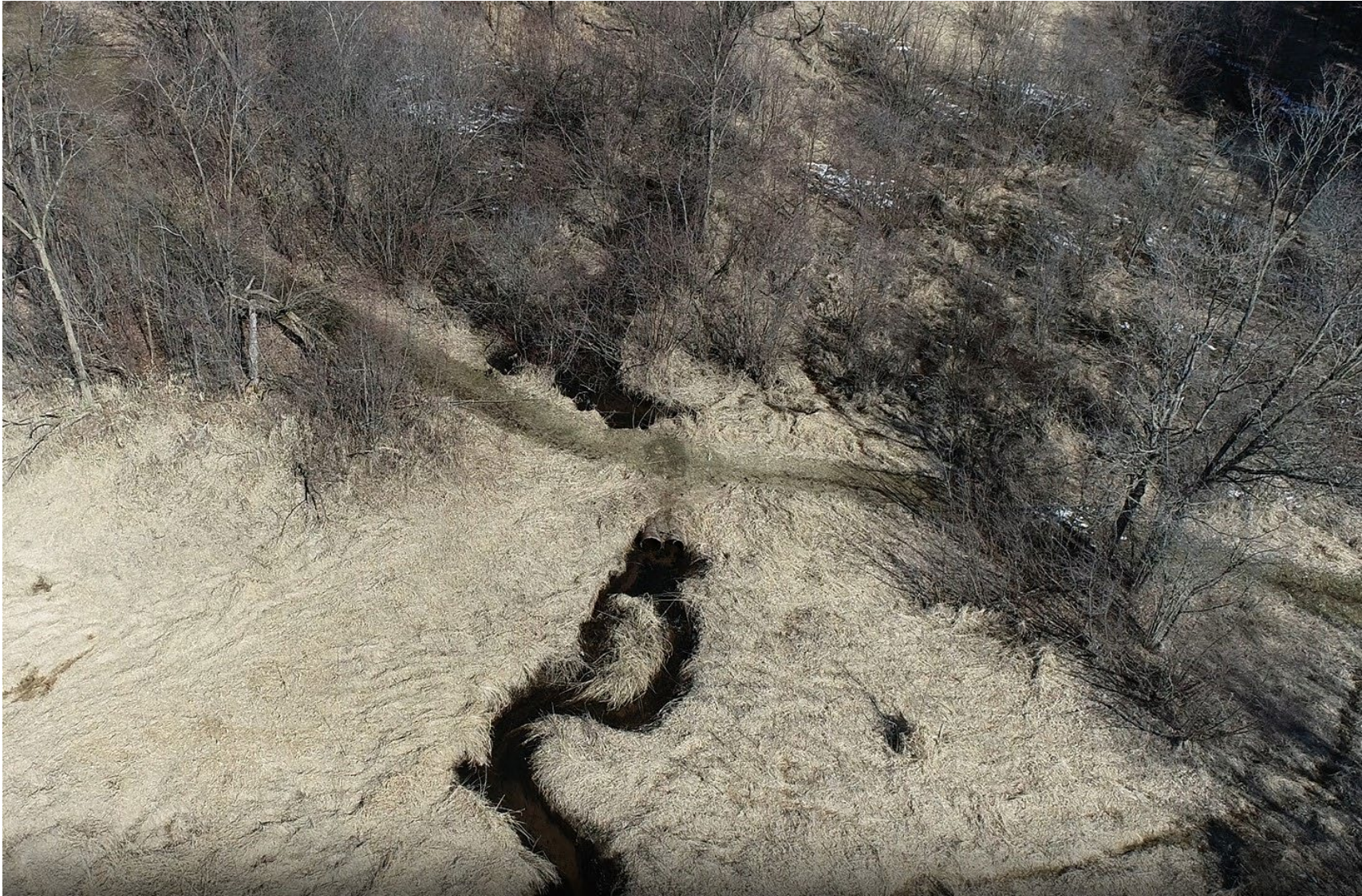
Twin culverts under a trail crossing downstream of 110 th St
