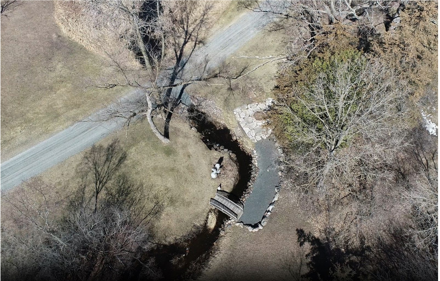
Driveway crossing and small foot bridge over Brown's Creek just upstream of 110 th St
