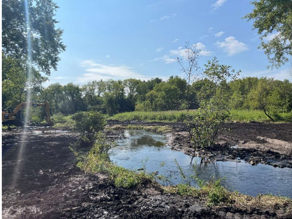
Picture above: Sods mats installed above brush/log toe.
