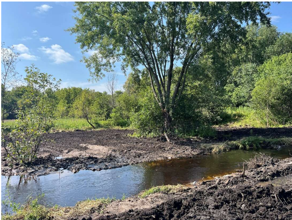
Picture above: Rock riffle installed (under high water conditions).
