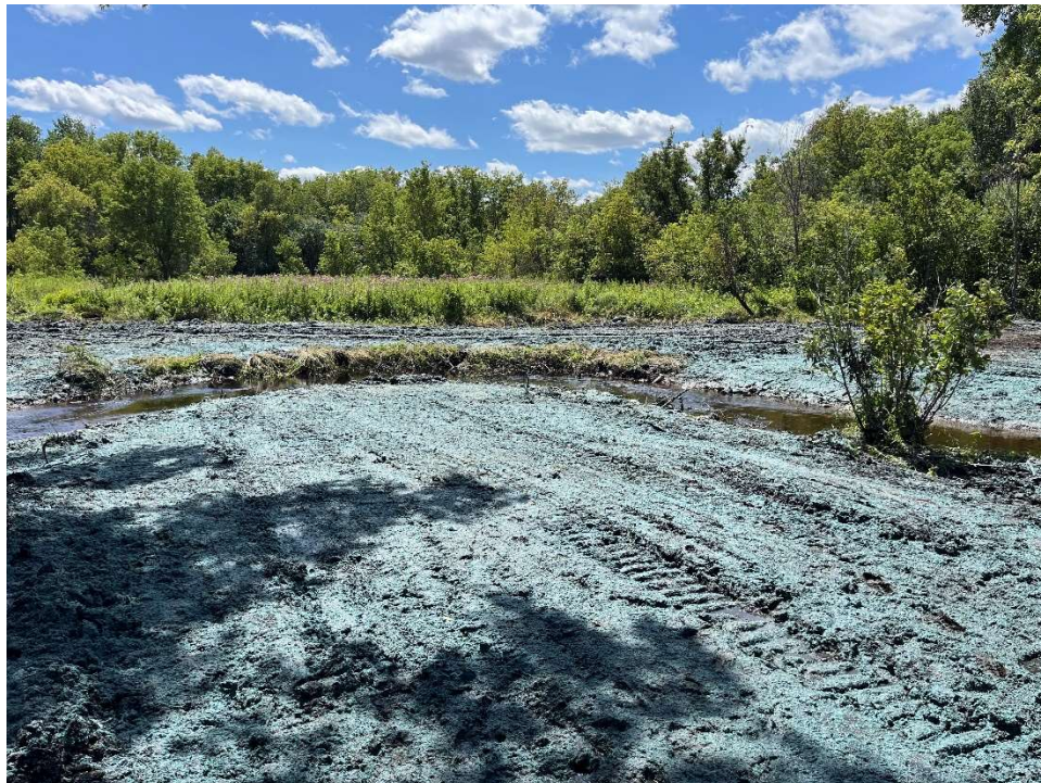
Picture above: Finished grade, area seeded and hyromulched.
