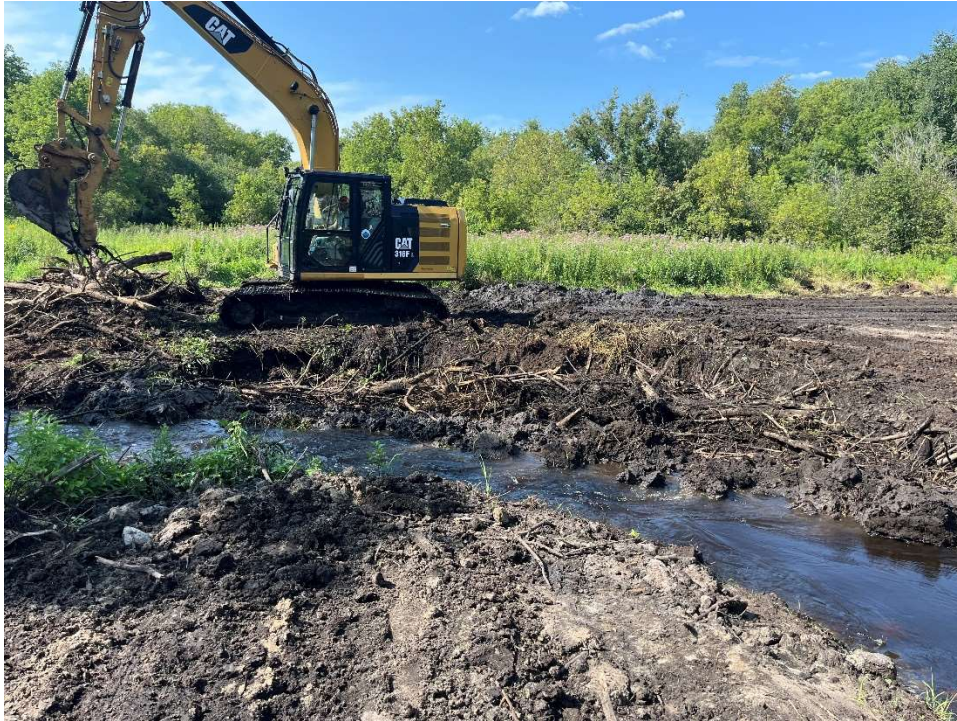
Picture above: Brush/log toe being installed.
