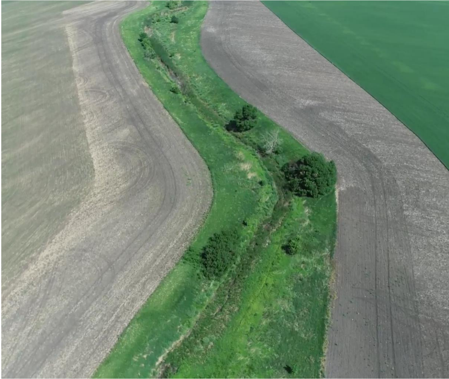
Site conditions before construction.
