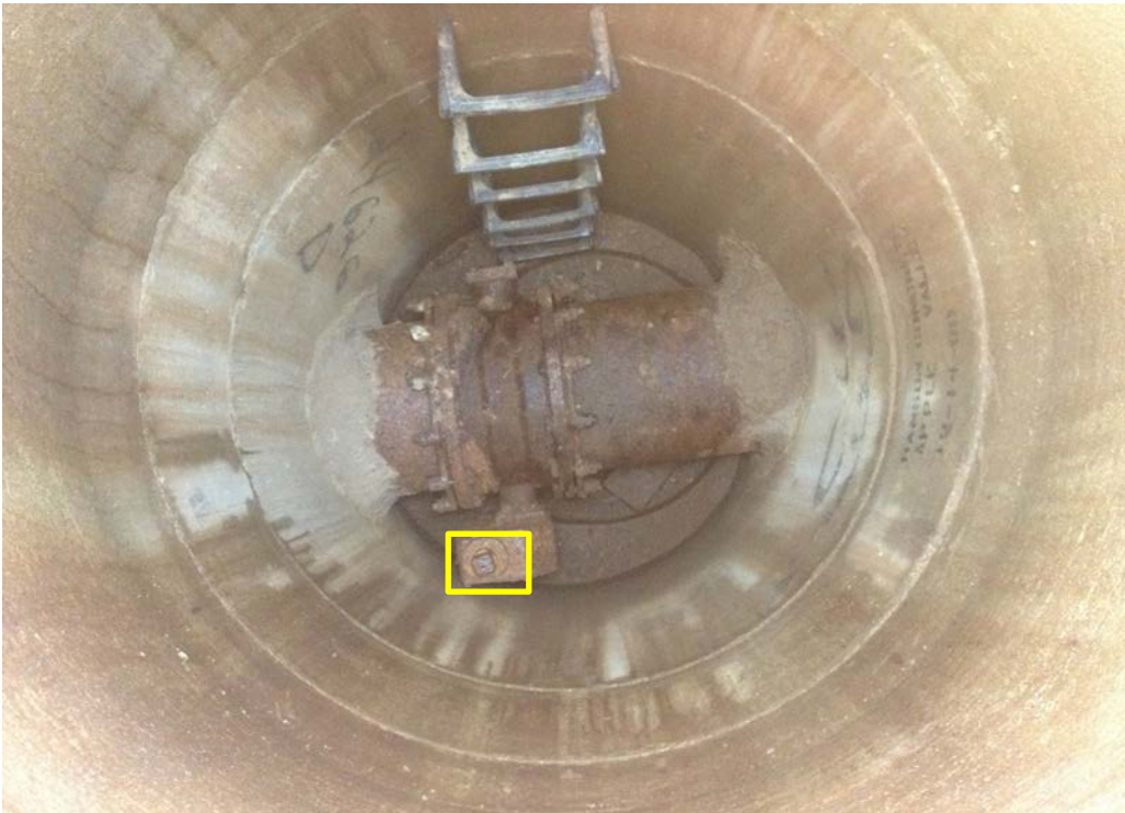
Figure 3. Goggins Lake gate valve nut (2" square nut highlighted in yellow). Turn counterclockwise to open the valve.
