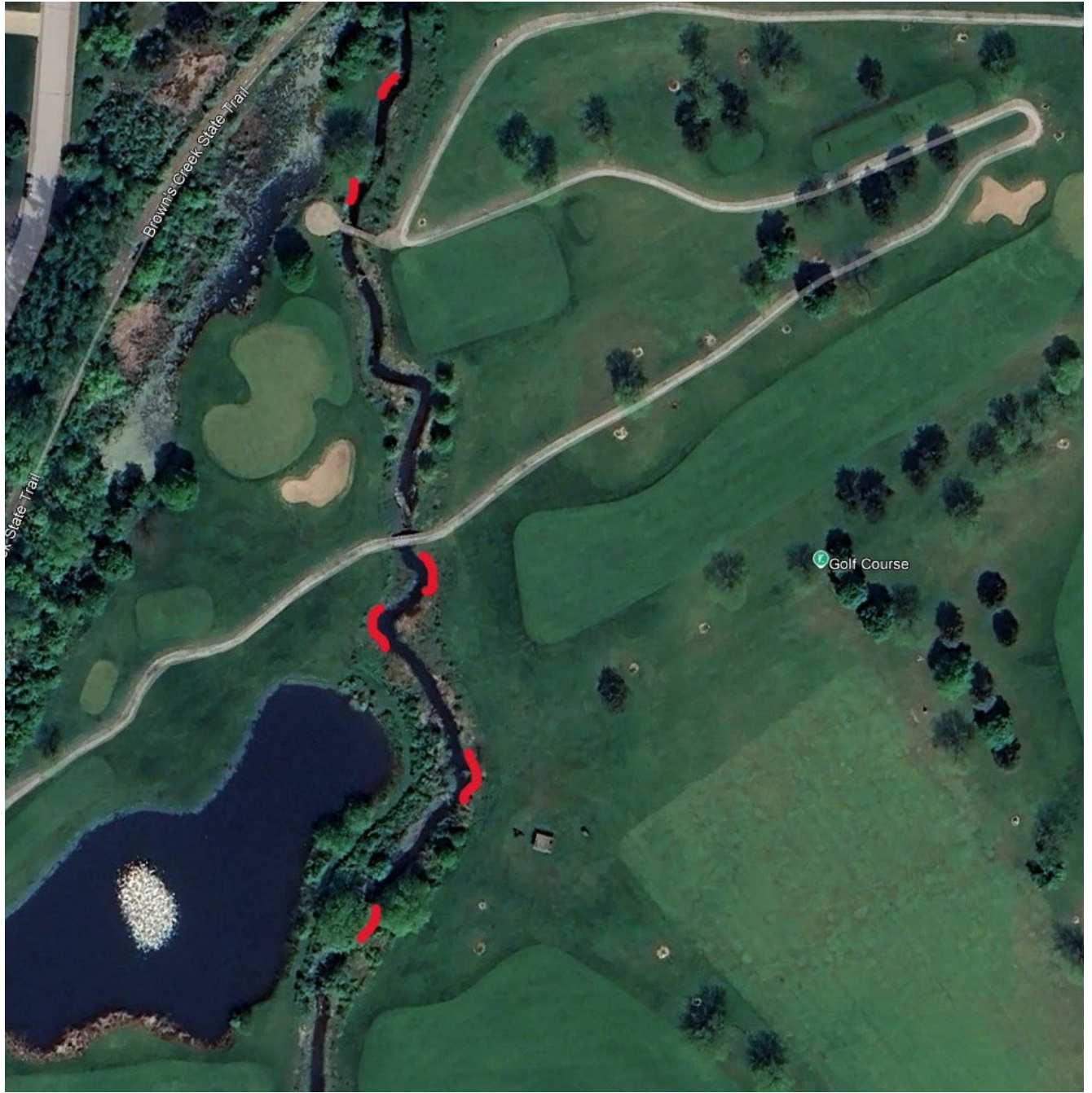
Figure 1. Proposed Brown's Creek bank repair sites (red lines) along the Oak Glen golf course.
