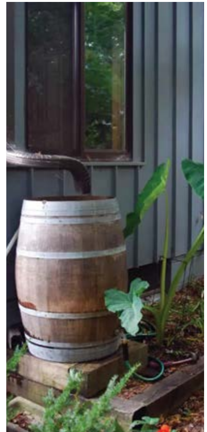
Using a rain barrel to capture water
