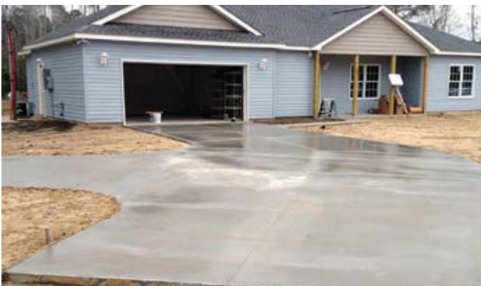
Adding impervious surface with a new driveway
