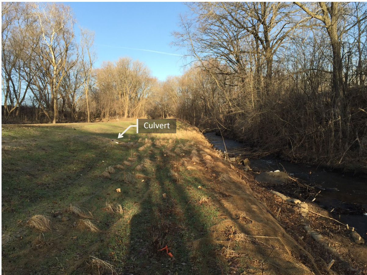
Figure 3. Site post-construction, showing primary area to be maintained and culvert location.
