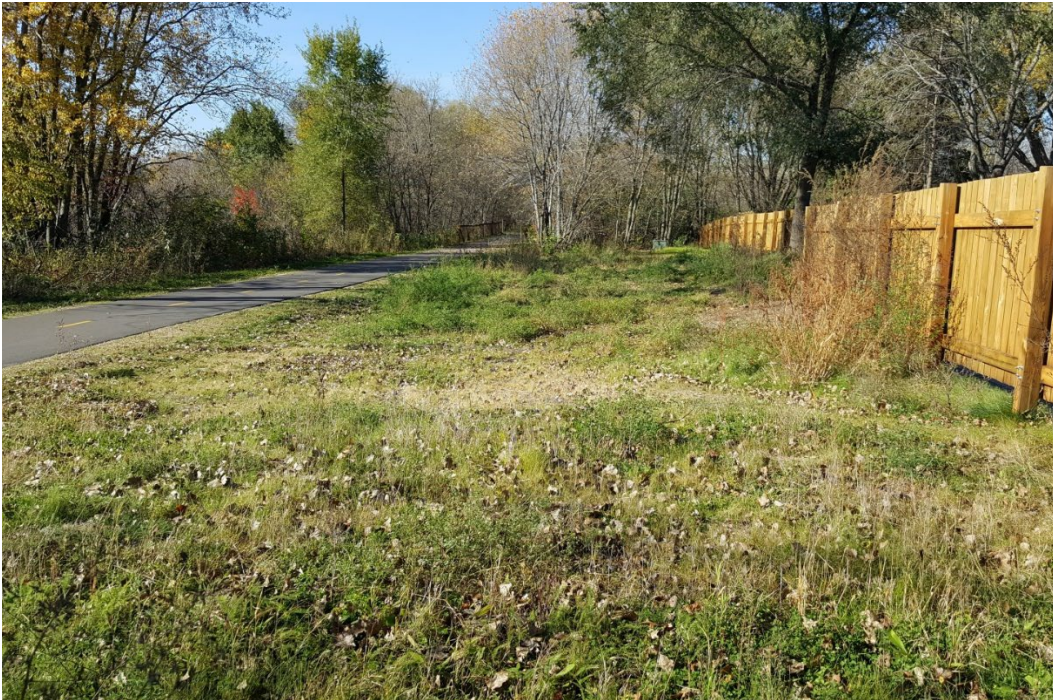
Figure 2. Countryside Auto Repair Water Quality Project looking west.
