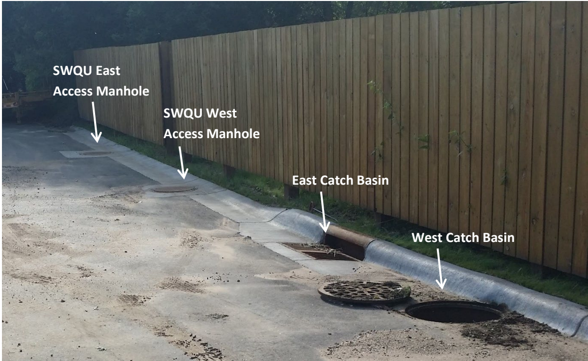
Figure 4. SWQU access manholes, catch basin locations.
