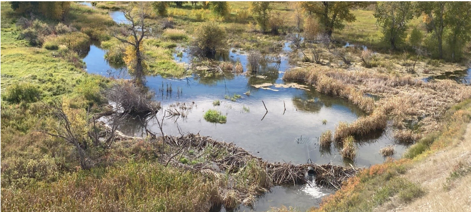
Figure 23: Example of an installed pond leveler in Montana. Photo Credit: Elissa Chott.
