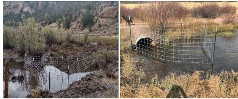
Figure 25: Exclusion fence installations are all site-specific and using the basic design principles, can be adapted by a trained professional for a variety of different waterways and needs. Photo Credit (left): Aaron Hall; Photo Credit (right): Elissa Chott.
