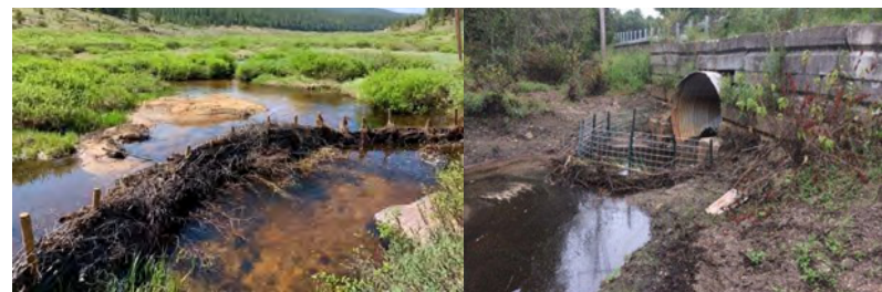
Figure 28: Diversion dams are site-specific. The same design principles can be adapted for a variety of different waterways and needs by a trained professional. Photo Credit (right): Jackie Corday (Colorado); Photo Credit (right): BeaverInstitute.org.
