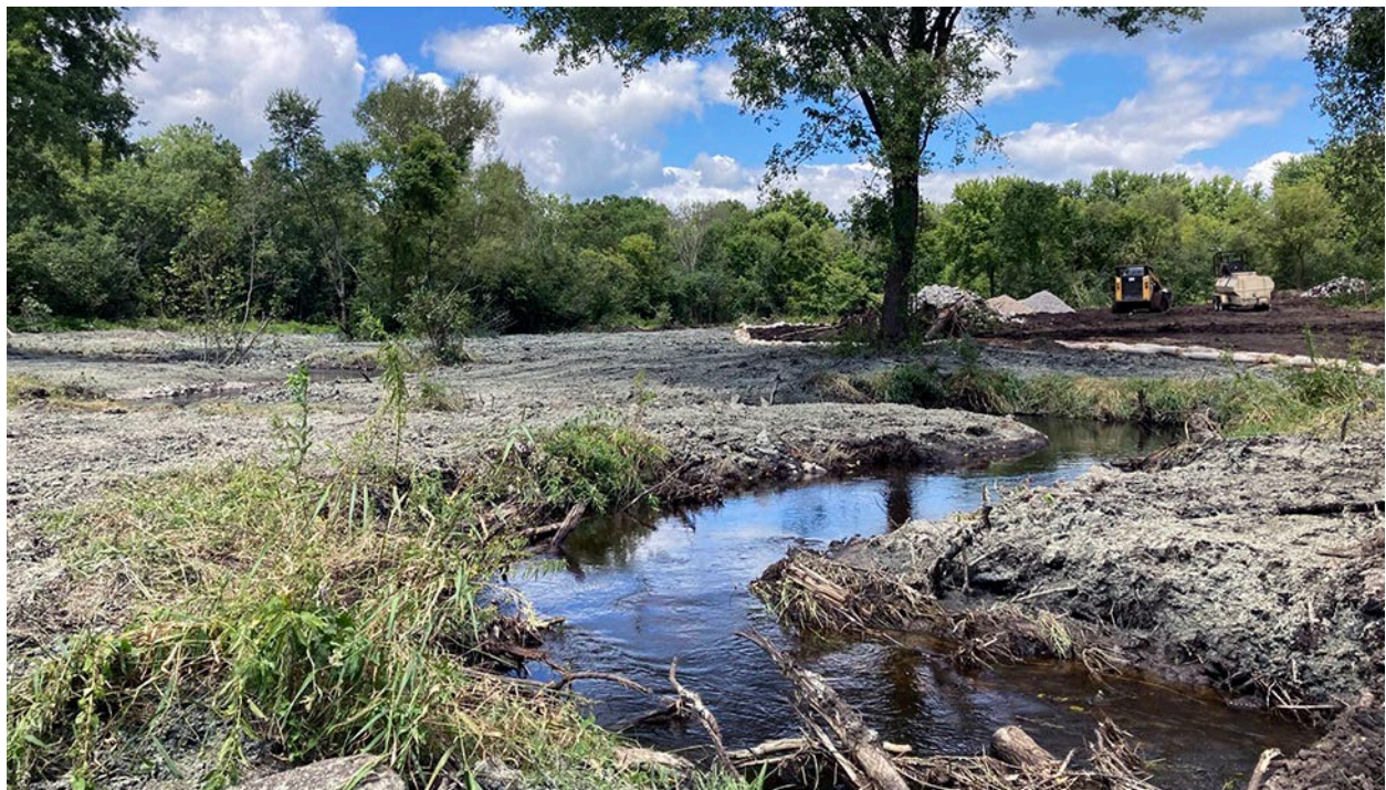
Brown's Creek restoration work completed in 2024 to address streambank erosion, among other concerns.
