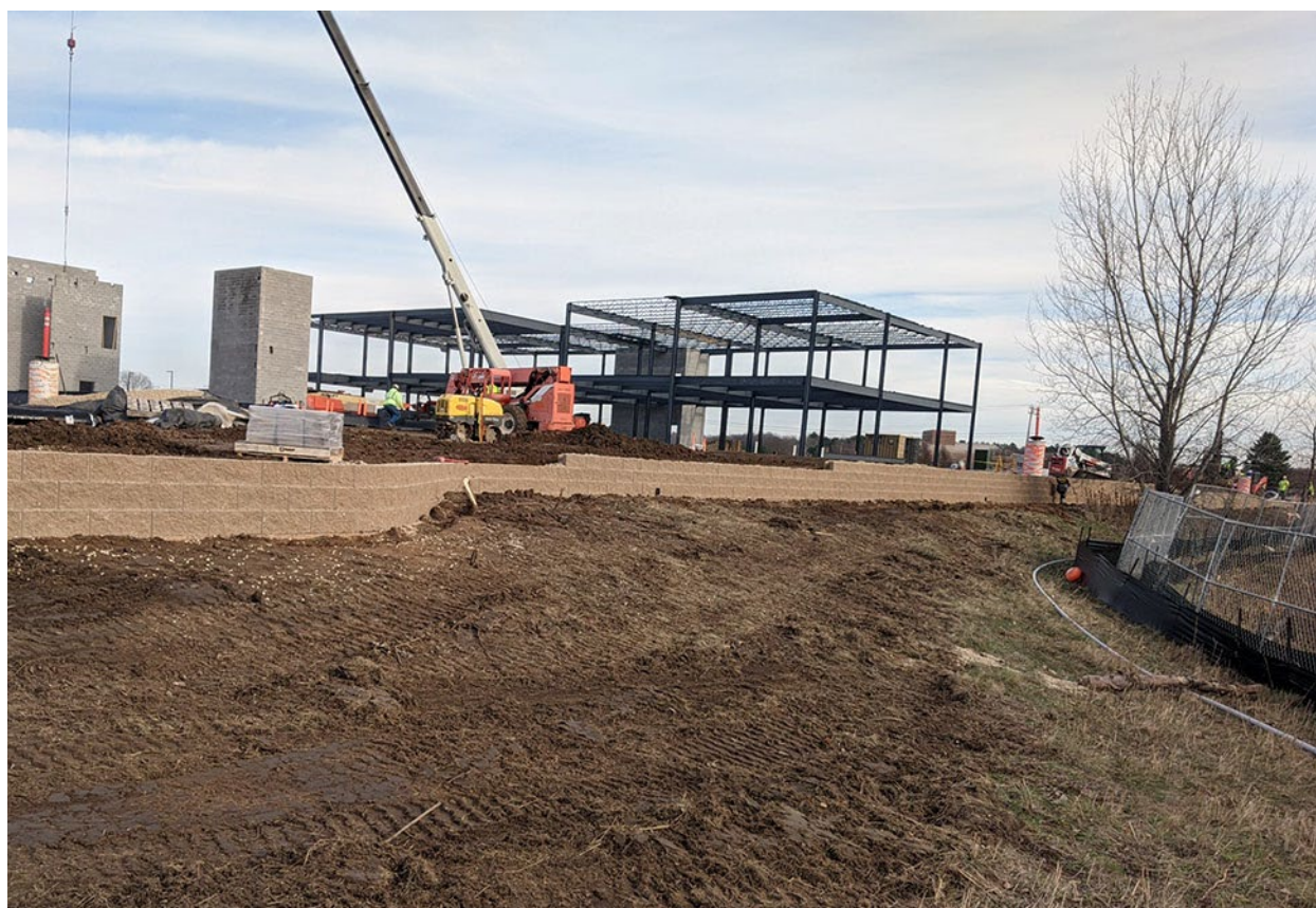
A permitted construction project in the watershed in 2025 using erosion control best management practices.
